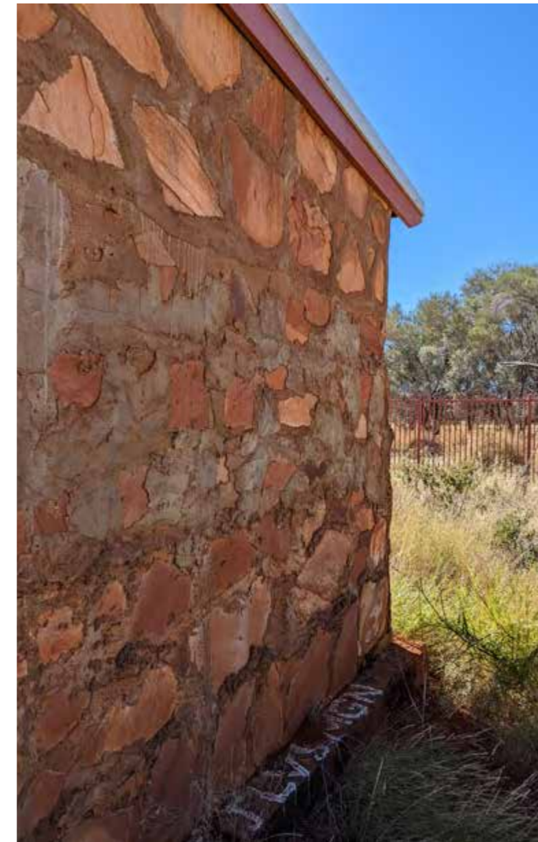
Warlukurlangu undertook the restoration of the Yuendumu Men's Museum that reopened in 2015. The building, located near the entrance to the town, was completed in 1971 and is built from stone quarried by local Warlpiri men from the hills above Yuendumu. The museum contains murals telling sacred stories that cannot be shown. Light is brought into the space via skylights, the most dramatic down the back wall (below).
