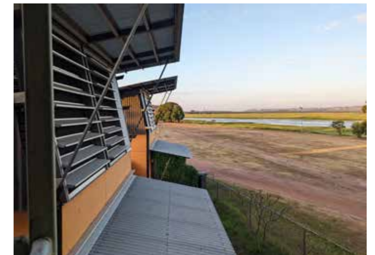
Built in 2016, the prefabricated accommodation units have a living space on the ground floor and a sleeping space above. Between the two units sits the bathrooms consolidating the services in the centre. They are naturally ventilated with screens and louvers that exposes them to the elements. They are currently not fully functioning.
