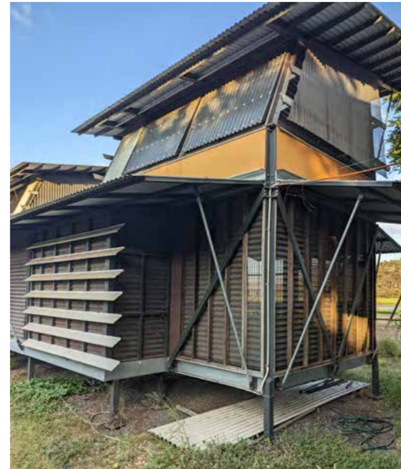
Built in 2016, the prefabricated accommodation units have a living space on the ground floor and a sleeping space above. Between the two units sits the bathrooms consolidating the services in the centre. They are naturally ventilated with screens and louvers that exposes them to the elements. They are currently not fully functioning.
